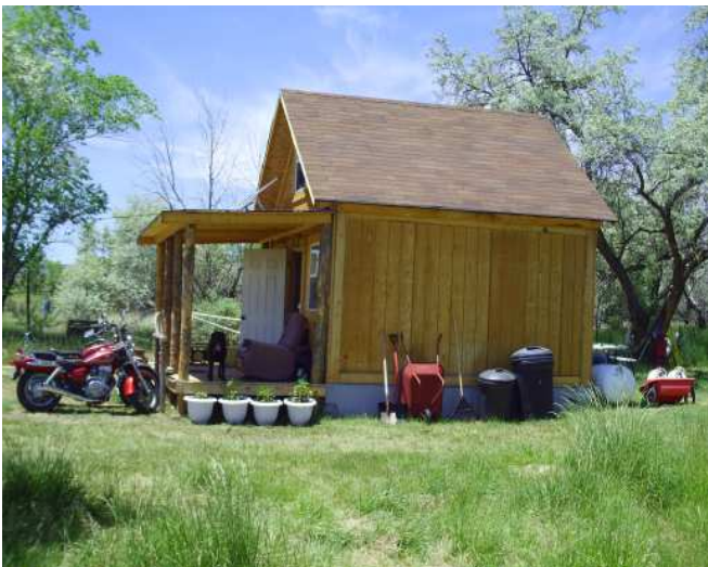
Side view of cabin and propane tank
