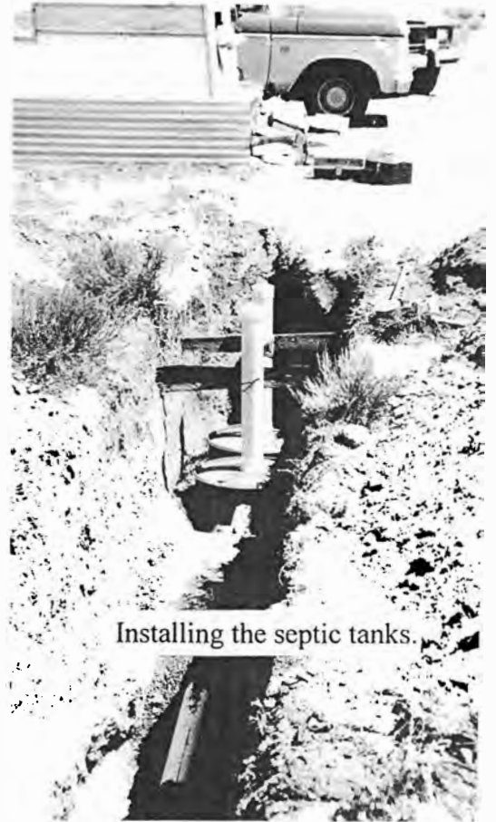
Septic barrels when first placed in holes.
