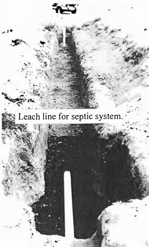
Installing the leach line.
