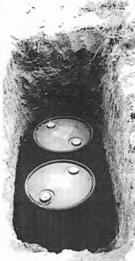
Septic barrels when first placed in holes.
